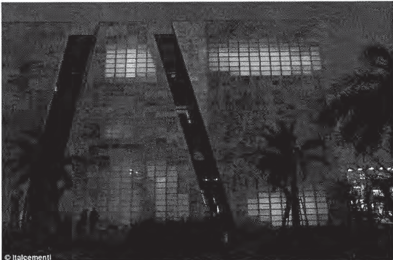
Architectural triumph: The Italian pavilion at last year's Expo in Shanghai is the only building constructed with 'transparent' cement to date
